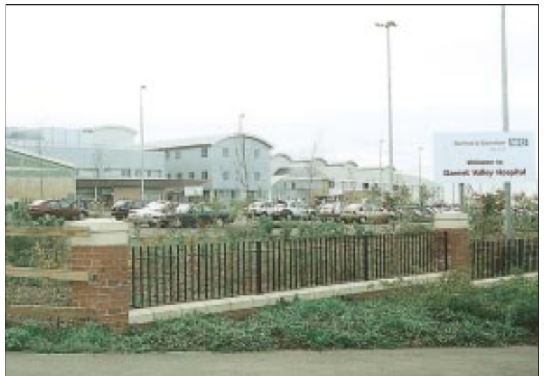
Darent Valley Hospital: nurses complained the design was not conducive to effective care
